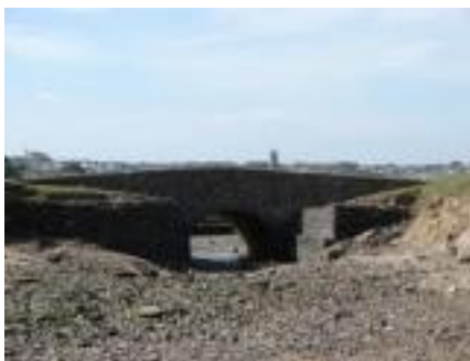
The small stone road bridge
